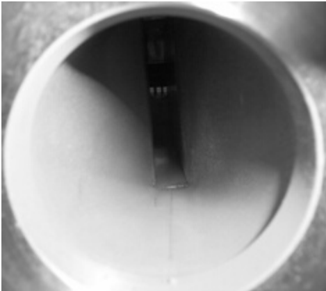
Figure 14: Measurement Conduit after Dusting
